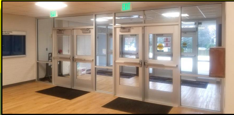
Completed Installation of Secure Entry Vestibule
