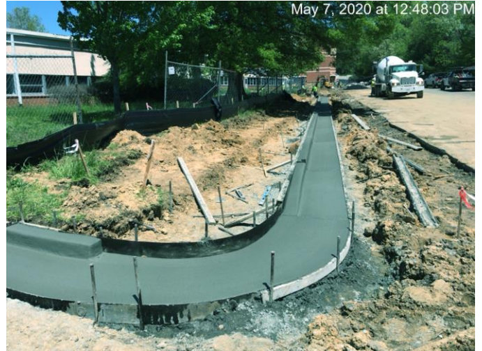
Site work – relocating sidewalk and shift lot
