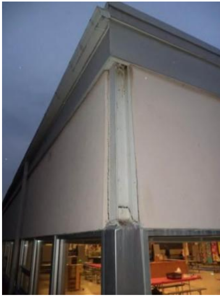
Figure 5: Exposed structural steel column @ Cafeteria.
