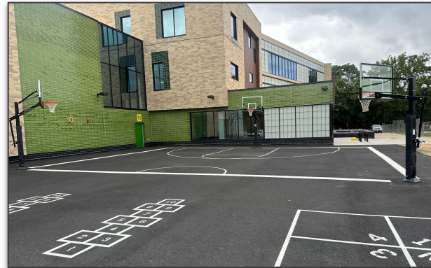
Douglas MacArthur Elementary School
