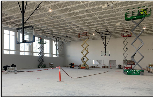
The High School Project: Minnie Howard Redevelopment
