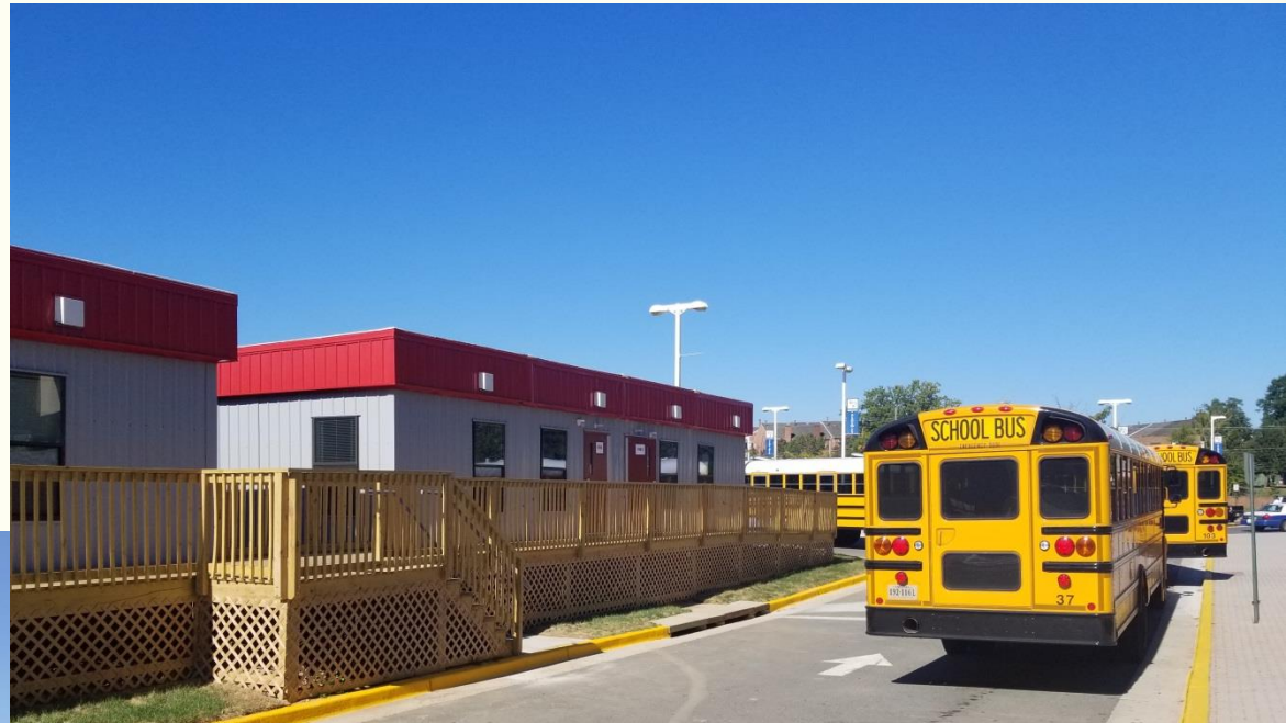
TC Williams: 6 Classrooms
