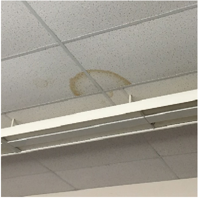
Figure 20 Ceiling Stains
