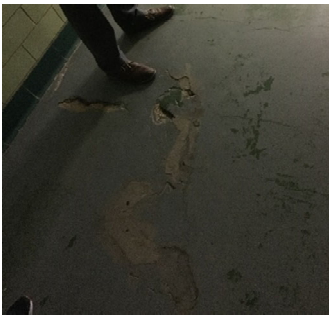
Figure 7. Floor slab and sub-structure in locker room corridor
