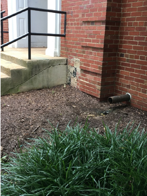
Figure 3: Crack on the entrance steps
