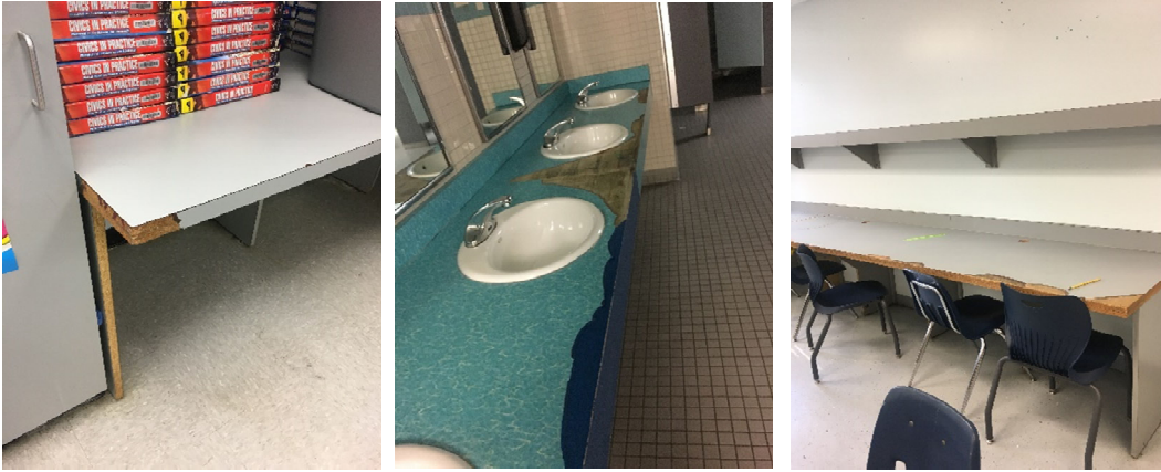
Figure 8 Aged Furniture and Counter Laminate
