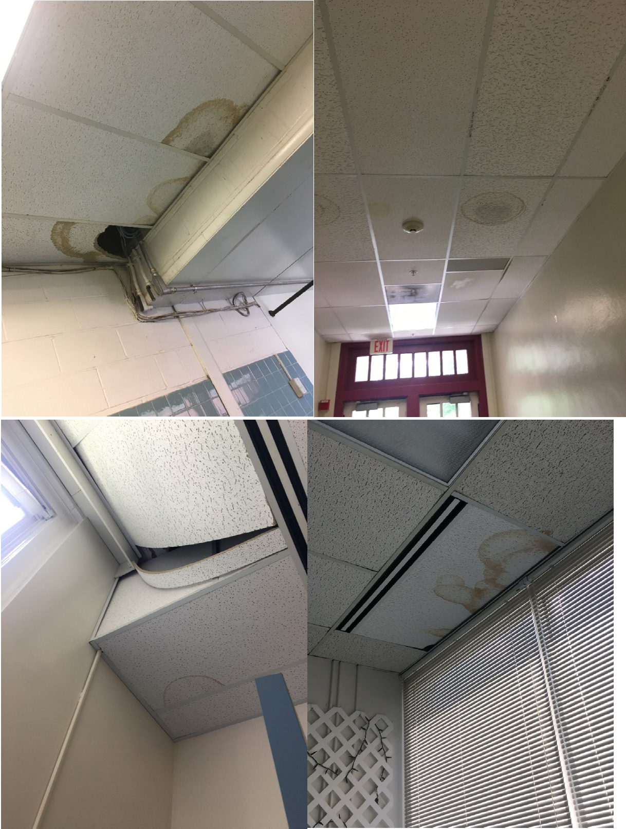
Figure 5: Ceiling stains
