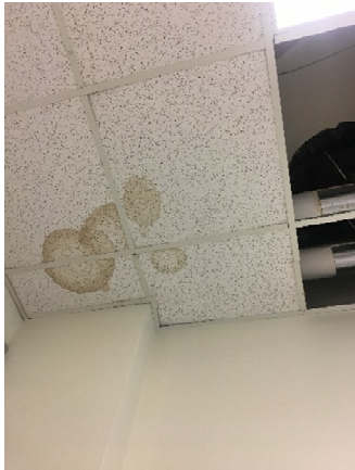
Figure 6 Ceiling Stains
