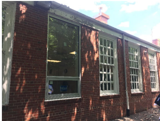
Figure 4 Stormwater Drains at Window Edge
