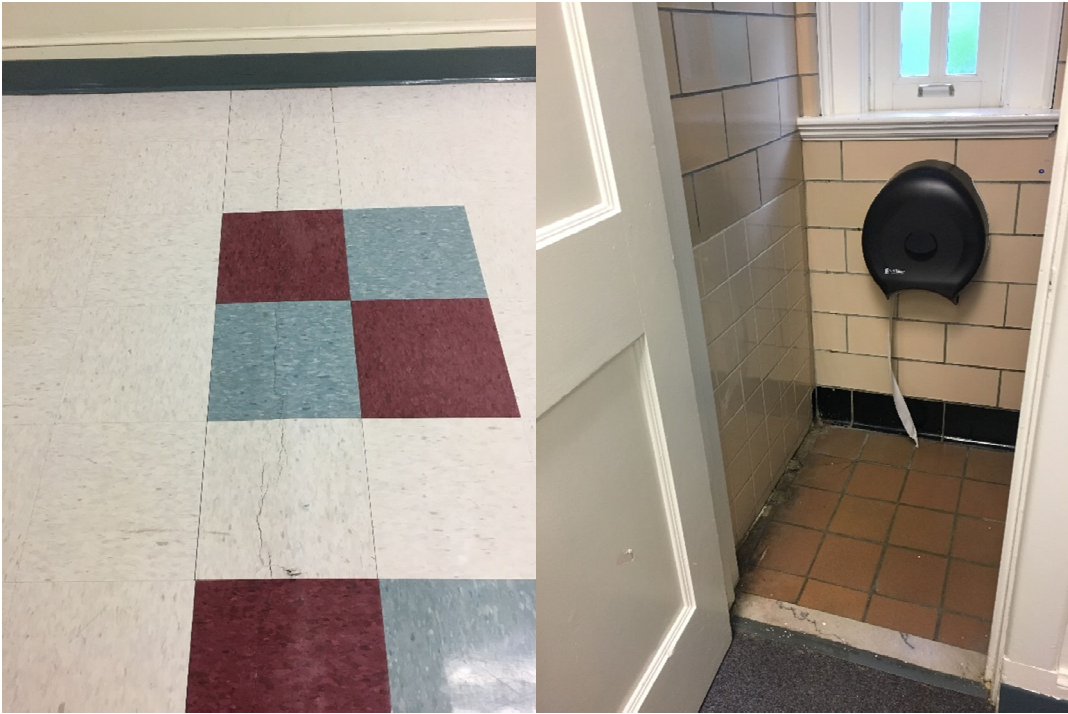
Figure 6: Cracked floor
