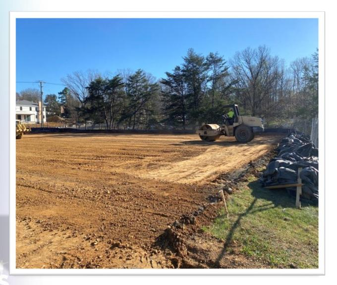
**Progress through Q3:** Contractor mobilized on-site and work commenced with the removal of existing tennis court surface and underlying sub-base materials. Excavation lowered the subgrade to the design elevation and the soils were amended with soil cement to achieve design compaction.
