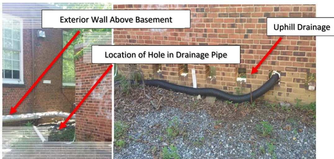
Photos 2 and 3. Drainage Downspout Above Basement Wall
