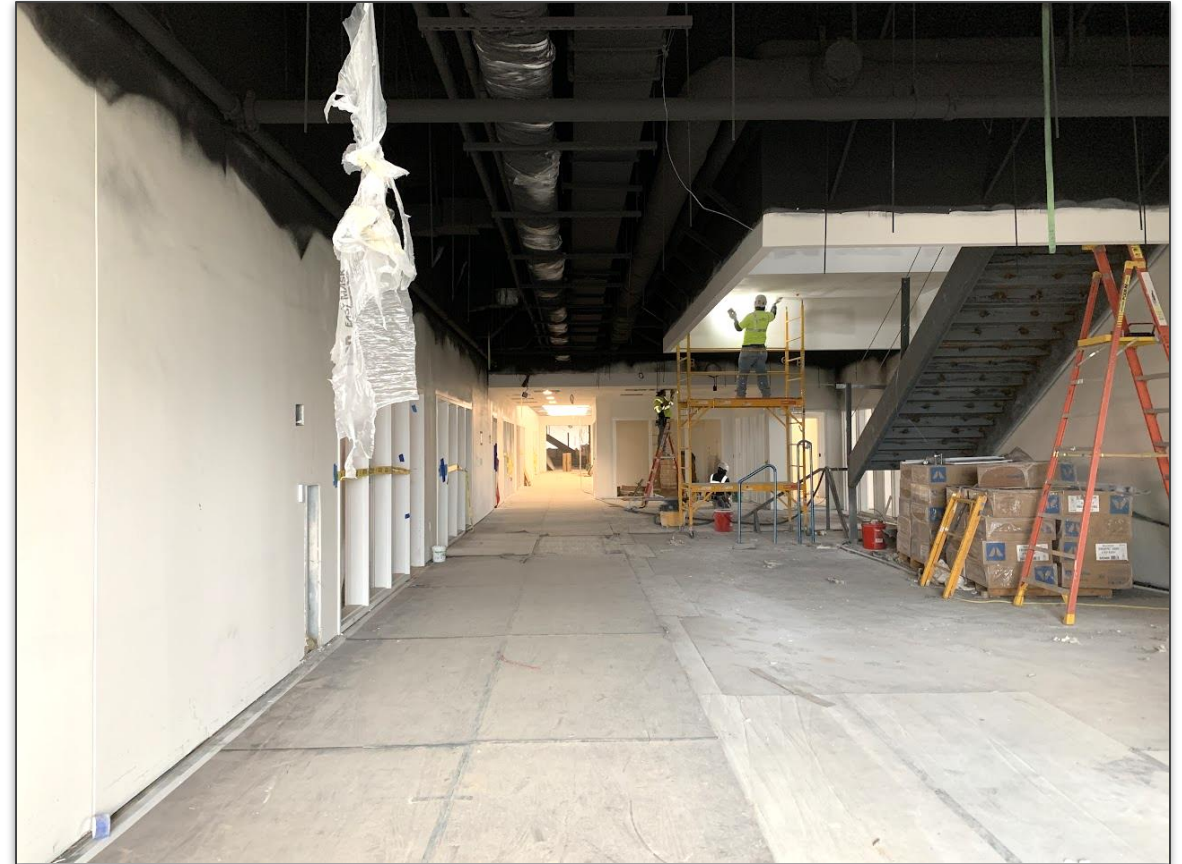
Area D Corridor
