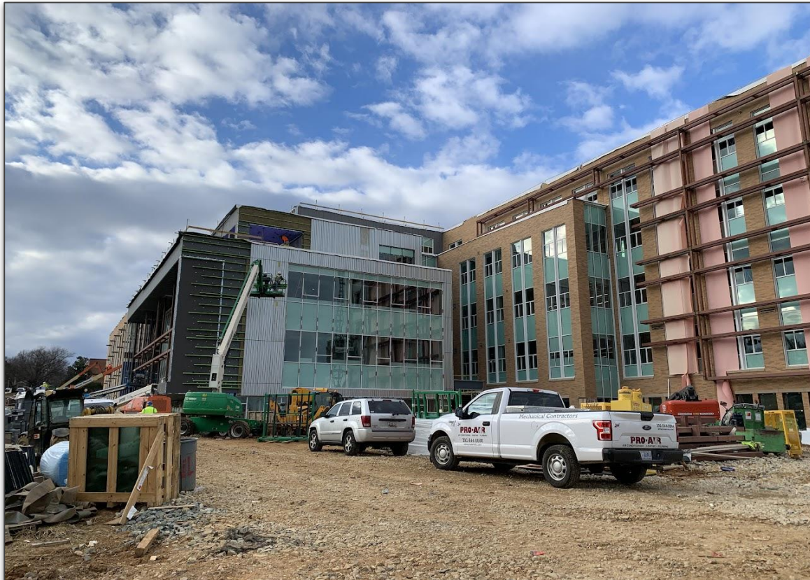
South Elevation- Facing Braddock Rd.
