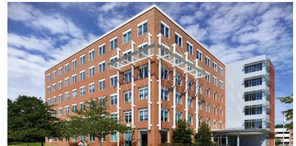
Ferdinand T. Day Elementary School Adaptive Reuse of Office Building – Elementary School & Future ACPS Admin
