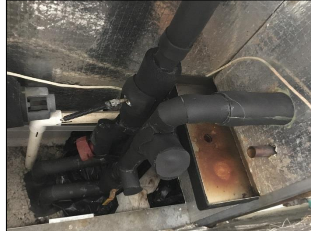
New fan coil unit pipe insulation.
