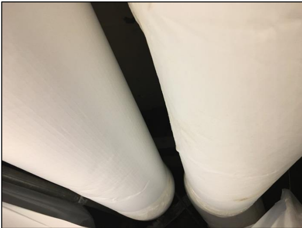
New dual temp pipe insulation.
