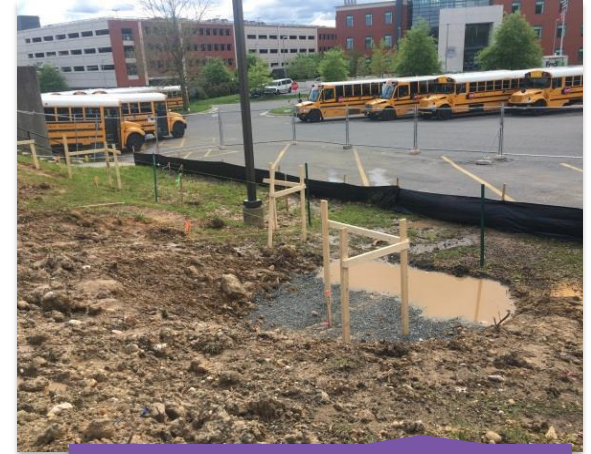
Erosion Protection (Silt Fence)
