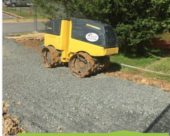
Grading for New Entrance
