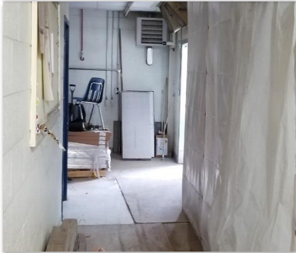
Loading Dock Hallway
