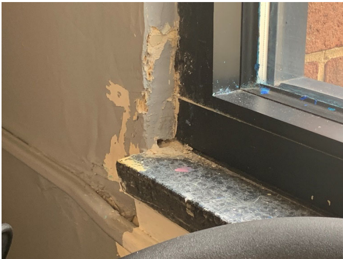
Figure 8: Paneling under the window pulling apart
