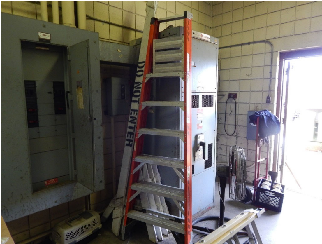
Figure 12: Panelboards and Transformer Exposed to Deteriorating Elements and Being Obstructed by Storage
