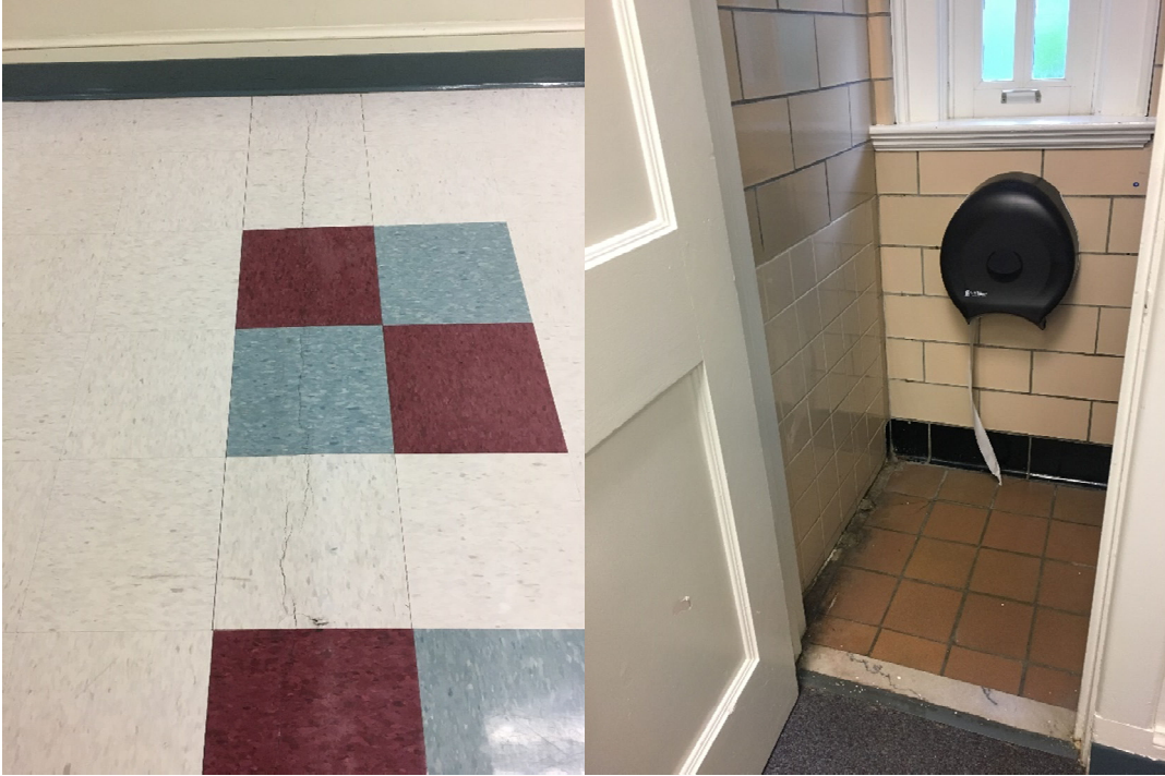
Figure 6: Cracked floor
