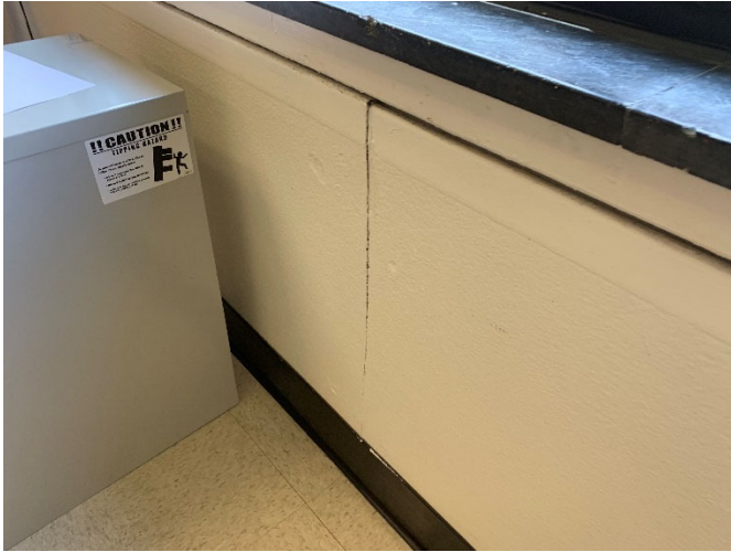
Figure 8: Paneling under the window pulling apart
