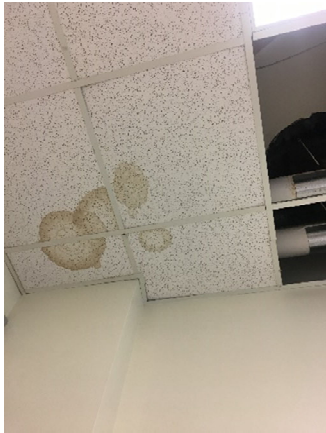
Figure 6 Ceiling Stains
