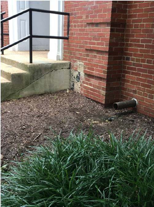
Figure 3: Crack on the entrance steps
