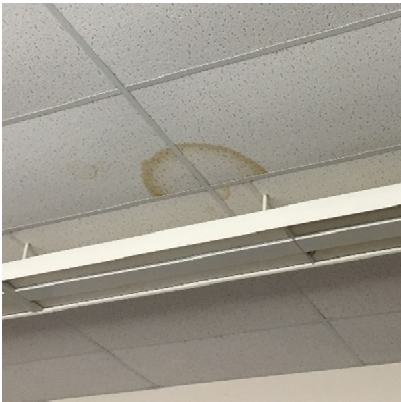
Figure 20 Ceiling Stains
