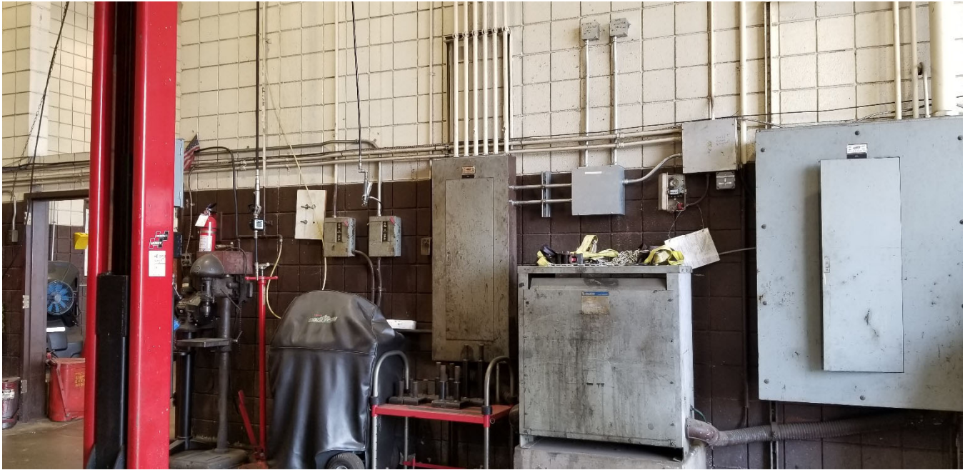
Figure 12: Panelboards and Transformer Exposed to Deteriorating Elements and Being Obstructed by Storage
