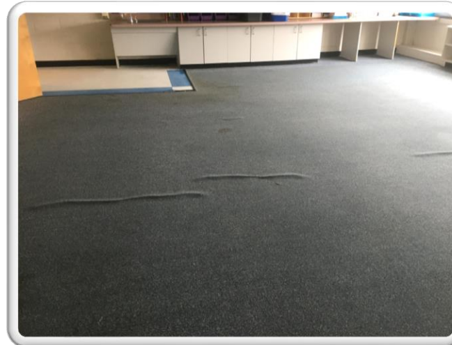
Lyles Crouch- Classroom Before and After
