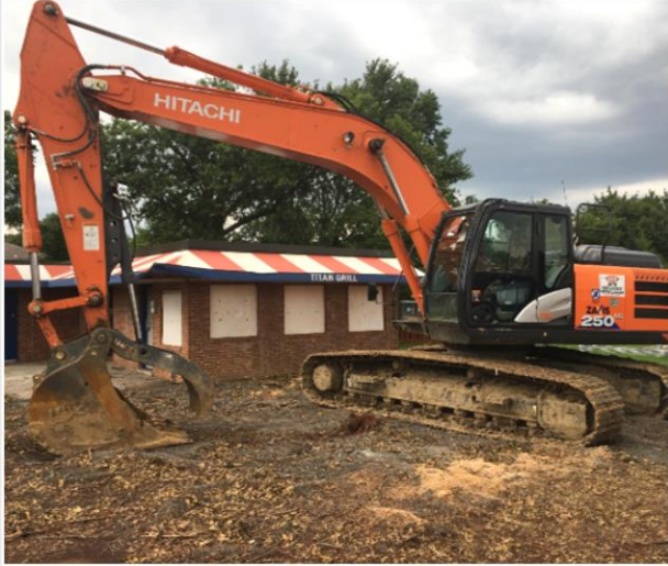
TC Williams Stadium Renovation
