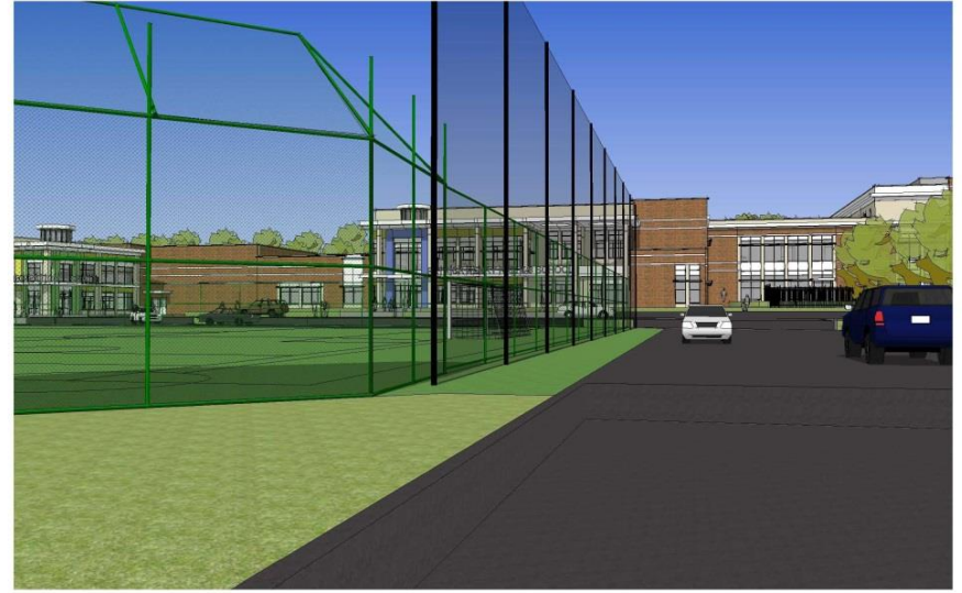
ENTRY DRIVE VIEW
