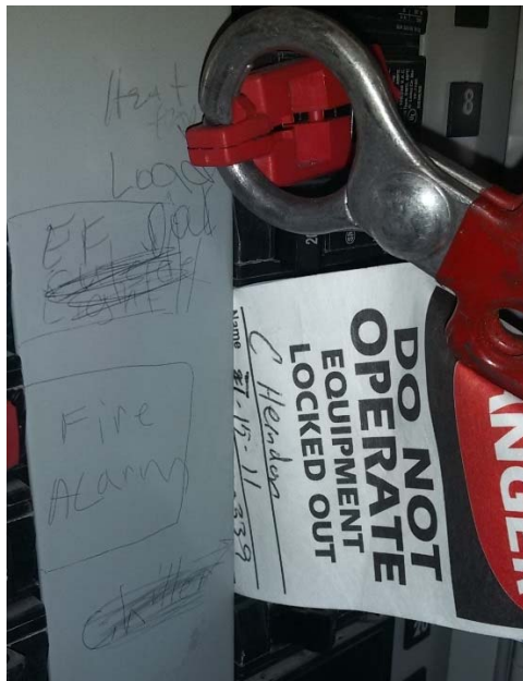
Photo 4. Lockout Device Applied at Samuel Tucker Elementary School
