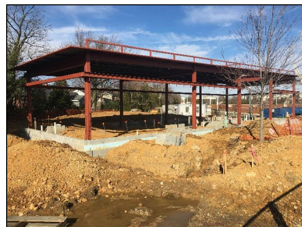
View of the restroom and storage building from the track.
