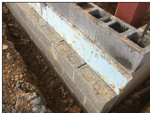
Foam insulation installed between concrete masonry unit courses.
