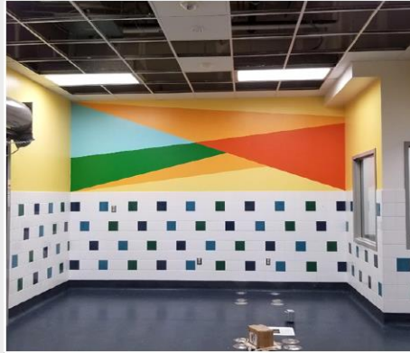
Kitchen and Servery Upgrades
