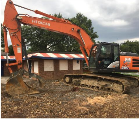
TC Williams Stadium Renovation
