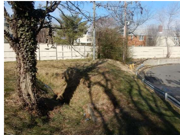
Image 2: Swale outfall to the Shopping Center
