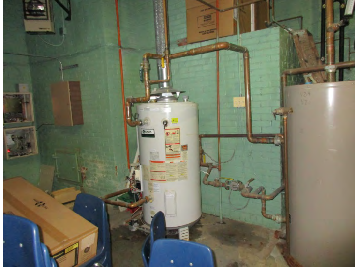
Single domestic water heater with supplemental tank
