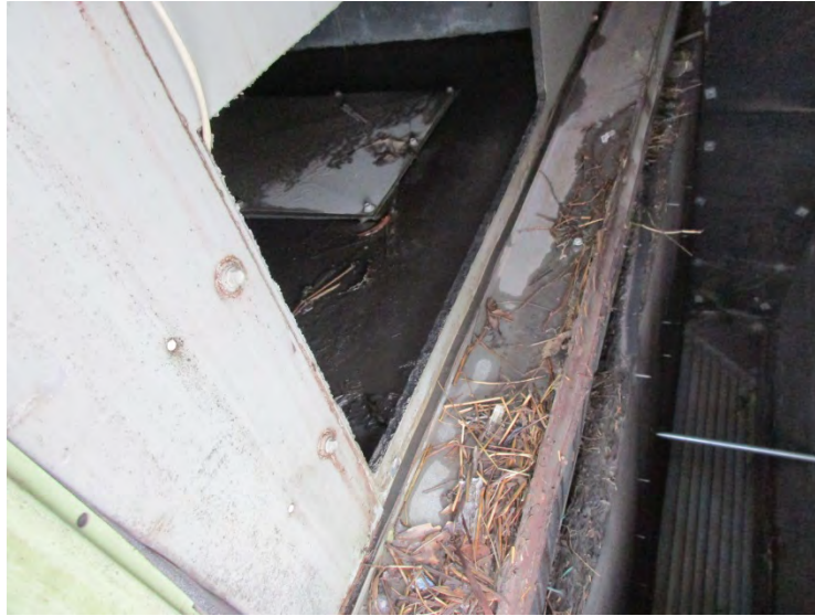
Debris found inside RTU-12.
