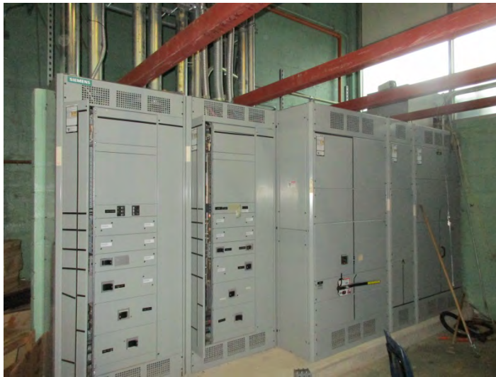
Electrical panelboards in boiler room in good condition.
