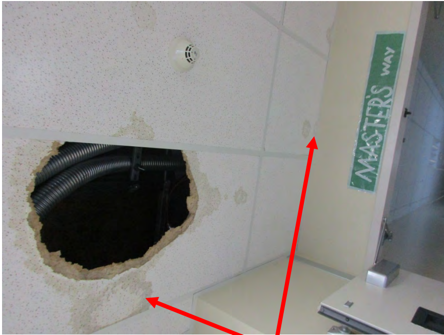
Watermarks found on damaged ceiling tiles.
