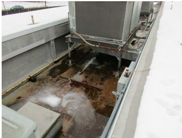
Pool of water surrounding RTU supports on roof.
