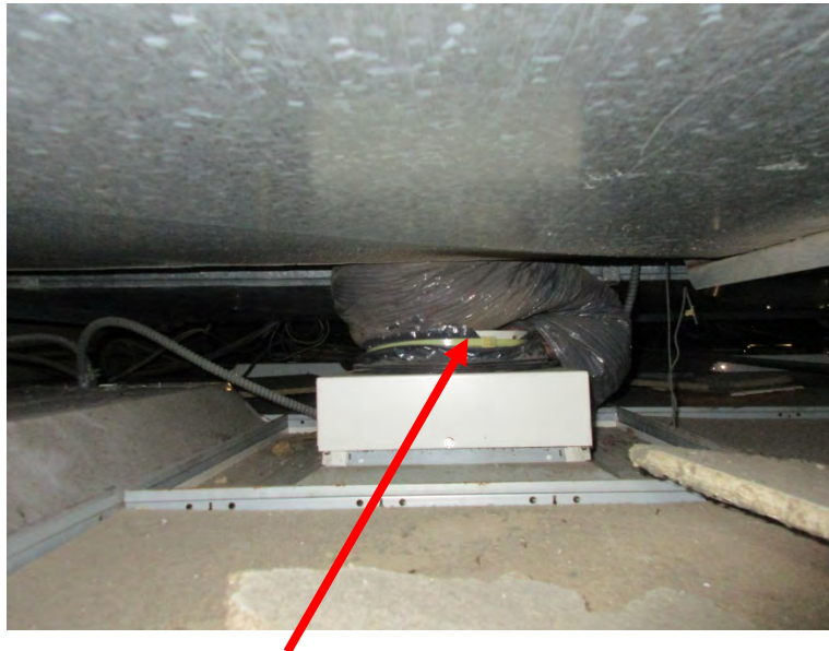
Broken supply flex duct above classroom ceiling.
