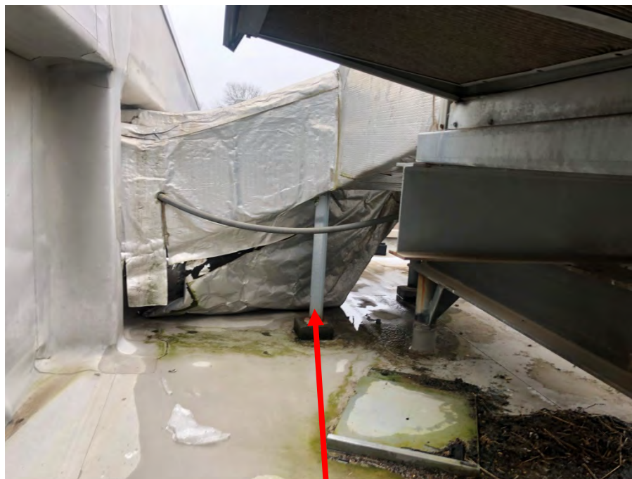
Insulation on exterior duct peeling off.
