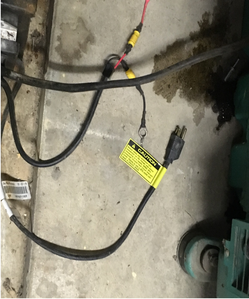
Photo # - 7. This picture is of the power disconnected from the emergency generator battery charger.
