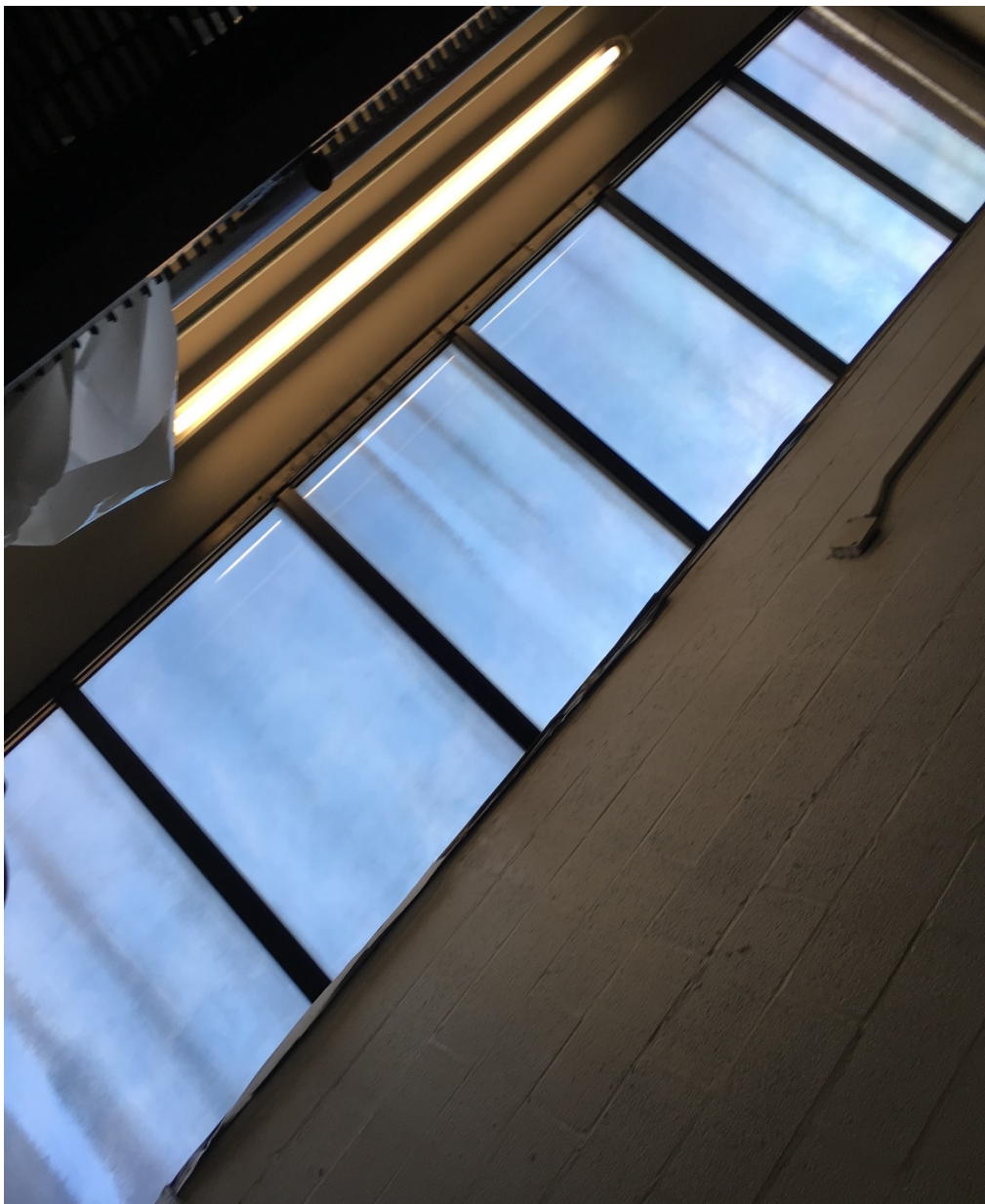
Photo – 12. This picture is of the firemen's equipment and gear room skylight which is leaking on the equipment.
