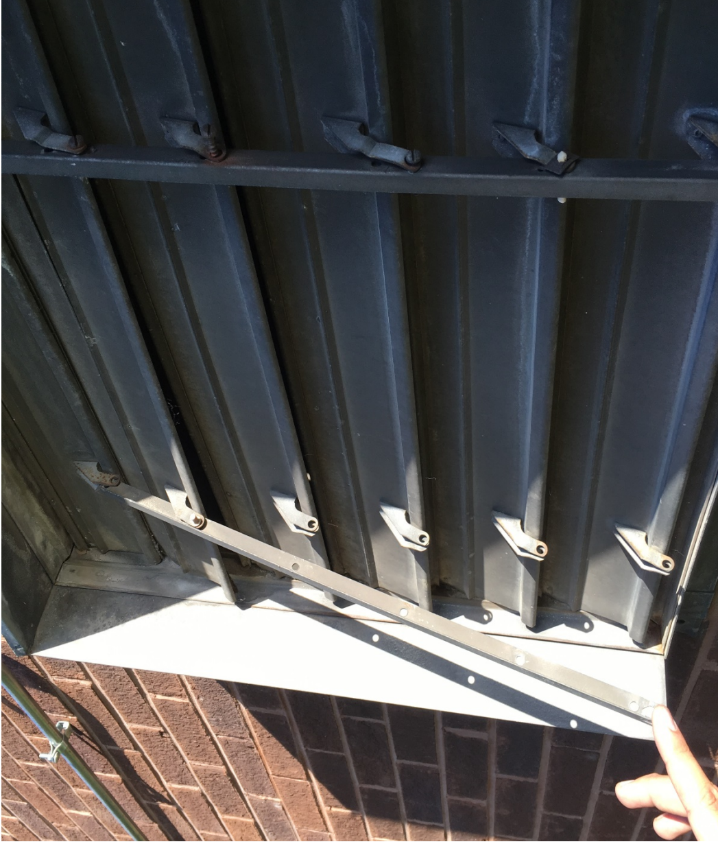
Photo # - 4. This picture is of the mechanical room exhaust fans backdraft damper which is falling apart.
