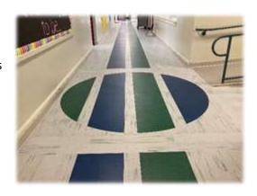
commenced with asbestos remediation and vinyl tile demolition at north and northwest hallways. The halls were leveled with Ardex and ready for return of students.
