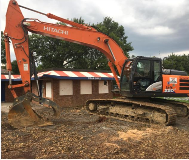
TC Williams Stadium Renovation
