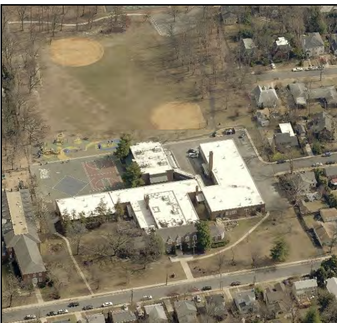
School site looking east across Cameron Mills Road. Note: This image does not reflect construction completed in Summer 2014.
