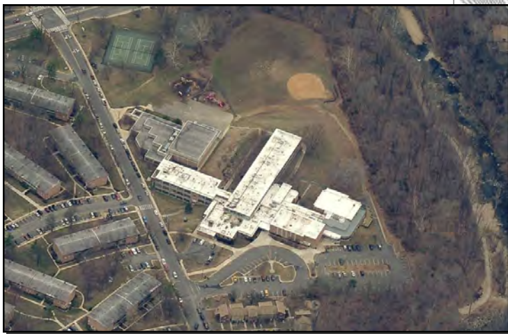
School site looking south across Sanger Avenue with Holmes Run on the right.
