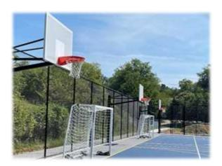
**Progress through Q4:** Construction continued with trenching and installation of perimeter under drains, installation of perimeter fencing, header curb and basketball support poles along with surfacing and game lines.
