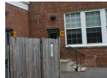
Photo #8 Typical Brick Deterioration and Repairs
