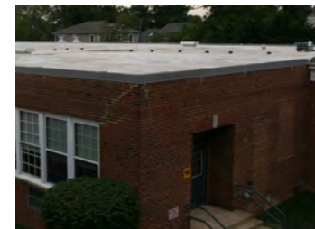
Photo #7 Typical Brick Deterioration and Repairs
