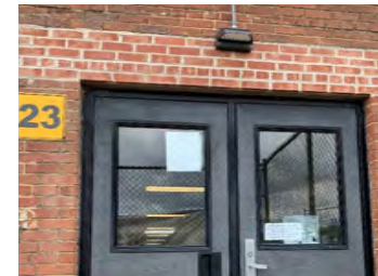
Photo #5 Typical Brick Deterioration and Repair
