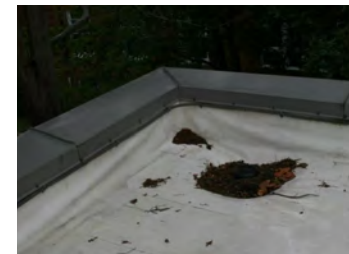
Photo #11 Clogged Roof Drain
