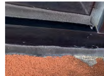
Photo #2 Typical EIFS Deterioration Bearing
