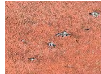
Photo #1 Typical EIFS Deterioration
