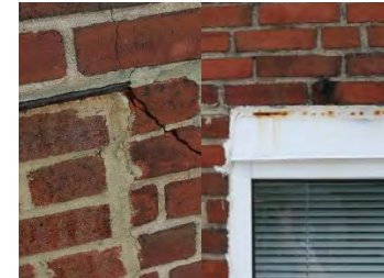
Photo #9, #10 Typical Brick Crack and Deterioration
