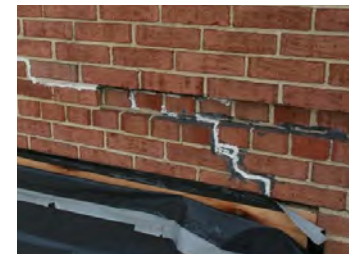
Photo #3 Typical Brick Crack and Repair Repairs
