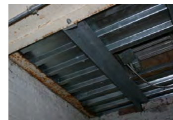
Photo #13 Rusted Steel Roof Over Mechanical Room Stair
