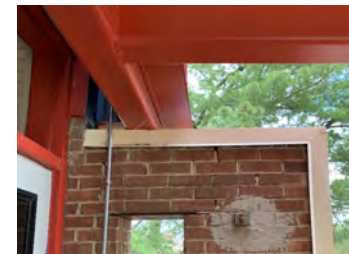
Photo #6 Brick Deterioration at Canopy Bearing
